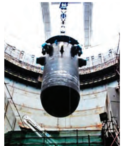
The reactor pressure vessel is cast from solid steel 20 cm (9 inches) thick.
