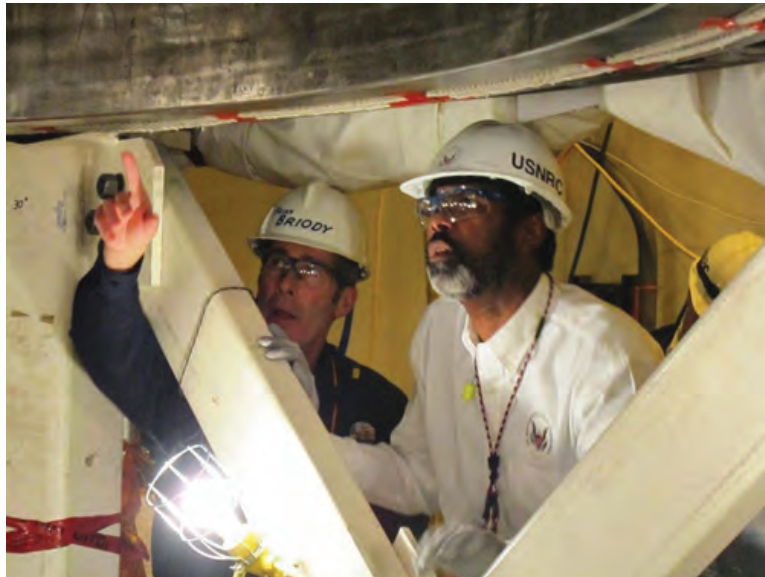
Regulators inspect the way nuclear power plants are operated and maintained.
