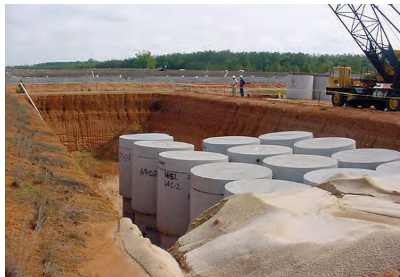
Low-level radioactive waste is stored in containers and covered with soil.
